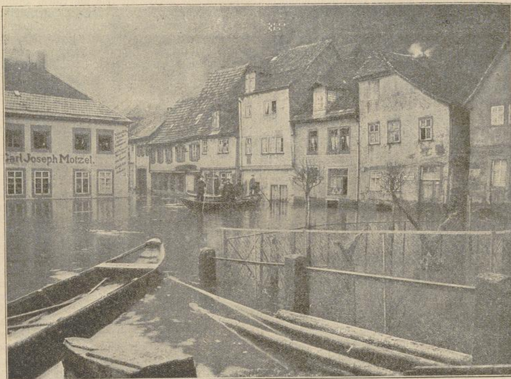
Hochwasser in Miltenberg am Main (Unterfranken).
